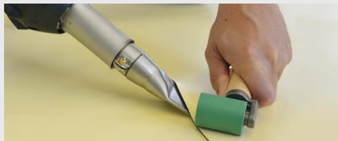
Overlap welding with the TRIAC ST
