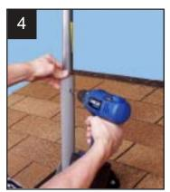
4) Remove Through Bolt. Insert antenna mast (customer supplied) into pipe. Insert optional Sleeve if using 1<sup>1/8</sup>-1<sup>1/4</sup>" mast. Drill a 5/16" hole through mast from each side using prepunched holes in pipe as guide. Insert Through Bolt and tighten securely.
