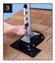
3) Plum Pipe to roof slope using the Plum Adjustment Bolt at bottom of foot. Use 7/16" wrench to securely tighten Plum Adjustment Bolt and Pivot Bolt.
