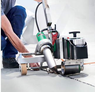
Welding modified bitumen
