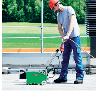
Overlap seam welding
