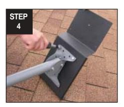
Install foot on deck plate using cap bolts
