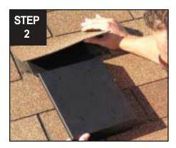
Before screwing base plate to roof, align both base & deck plate to assure shingles will fall into place
