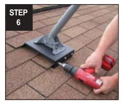
Use Tek Screws to secure deck to base plate
