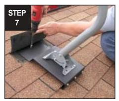
Install deck plate using trusshead screws, use small amount of roof cement under top shingle to secure
