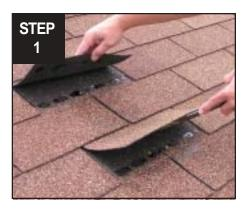
Locate truss with stud finder, lift shingles with prybar at dish location, do not lift middle row
