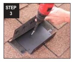
Install base plate with trusshead screws
